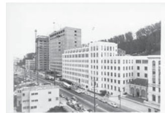
Moffitt Hospital under construction
