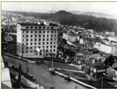
Aerial view showing the nurses' dormitory
