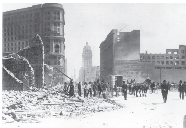
Down Market from Mason: This photo of the post-earthquake destruction on Market street, April 1906, reveals the site of the Donohoe Building (far left) which housed UC's dental clinics at the time.
