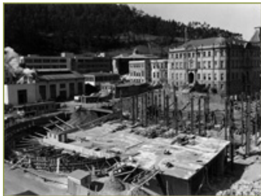
UCSF campus under construction, 1951
