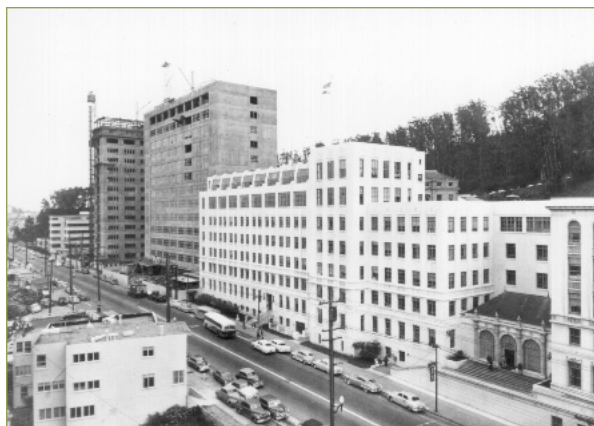
Moffitt Hospital under construction
