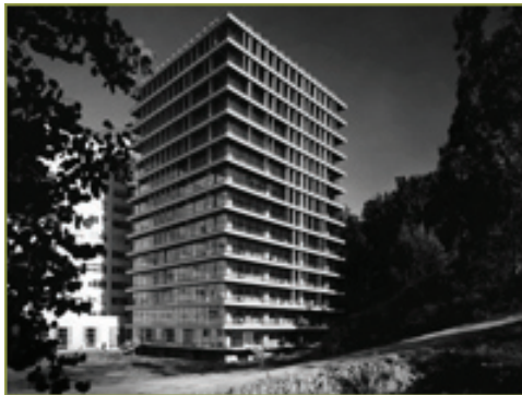
Health Sciences West tower, completed in 1966
