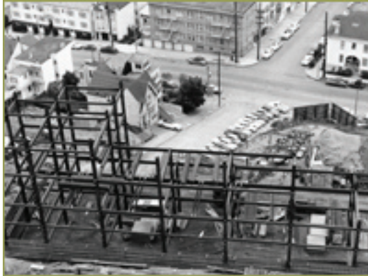
Construction of Millberry Union, 1956
