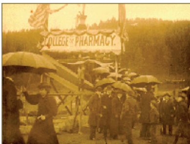
Laying cornerstone for the Affiliated Colleges on a stormy day, March 27, 1897.
