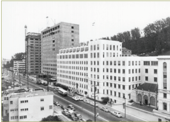
Moffitt Hospital under construction
