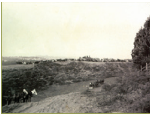
Grading the site of the Affiliated Colleges, August 29, 1895, John Tuttle, contractor.
