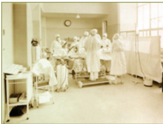
"Modern" operating room in the new UC Hospital, 1924.
