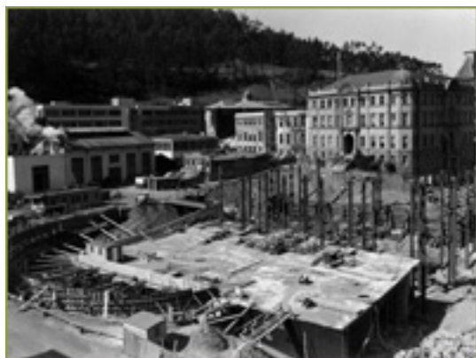
UCSF campus under construction, 1951
