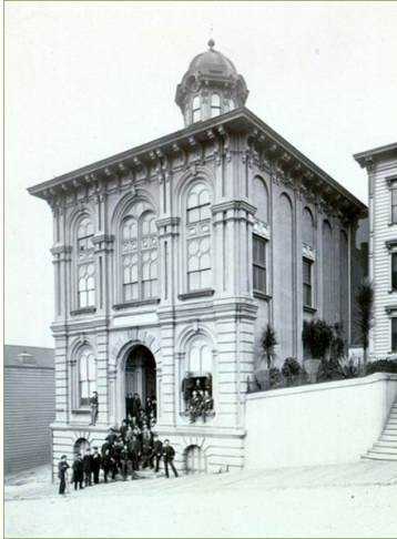
Closeup of Toland Medical Building; the three story City County Hospital is on the right. The hospital moved to its Portrero site in 1872, making clinical training more difficult for students who had to travel four miles for clinical sessions.
