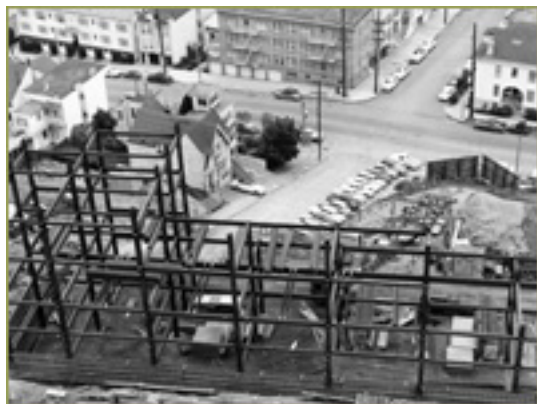
Construction of Millberry Union, 1956
