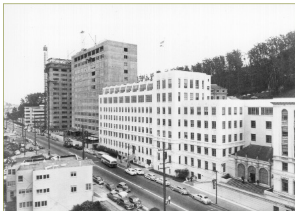
Moffitt Hospital under construction
