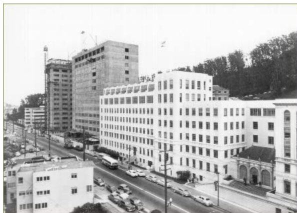
Moffitt Hospital under construction
