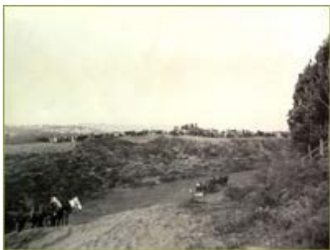
Grading the site of the Affiliated Colleges, August 29, 1895, John Tuttle, contractor.
