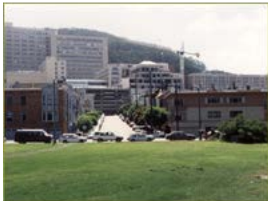
Construction of the UCSF Library (the building to the left of the crane)
