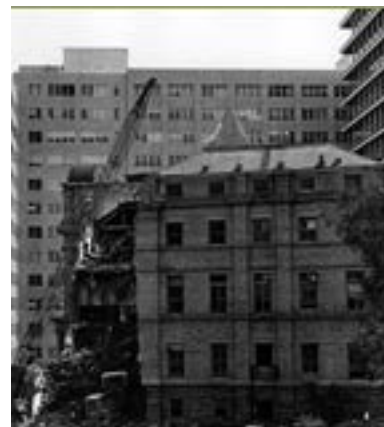
The old Medical School Building was demolished in 1967.
