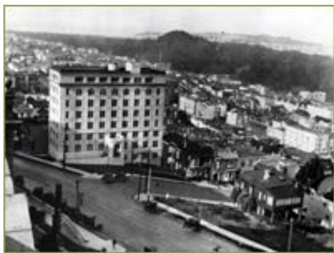
Aerial view showing the nurses' dormitory
