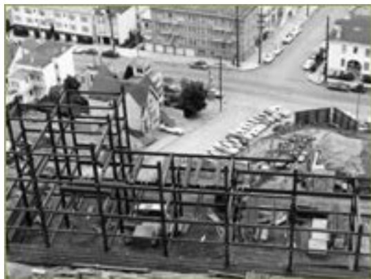
Construction of Millberry Union, 1956
