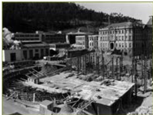
UCSF campus under construction, 1951
