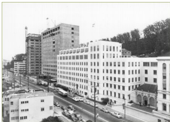
Moffitt Hospital under construction
