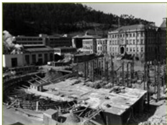
UCSF campus under construction, 1951
