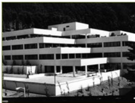
The new School of Dentistry building, completed in 1980
