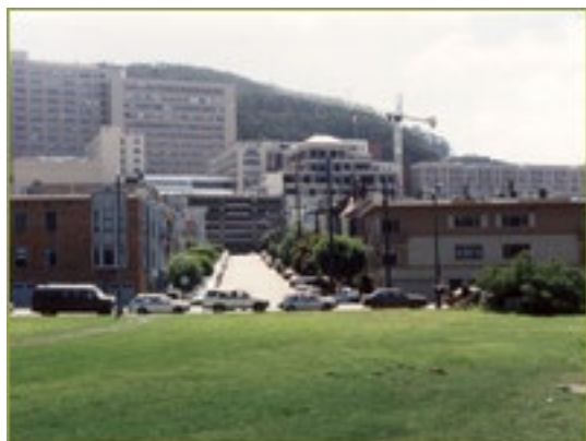
Construction of the UCSF Library (the building to the left of the crane)
