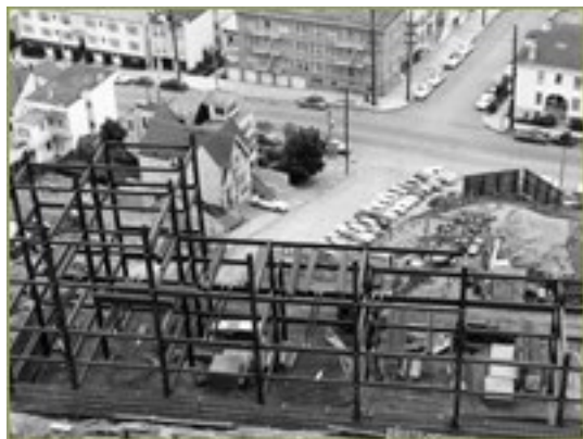
Construction of Millberry Union, 1956
