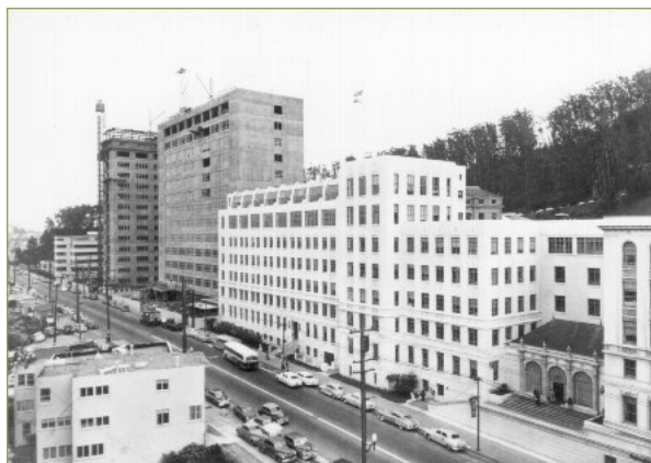
Moffitt Hospital under construction
